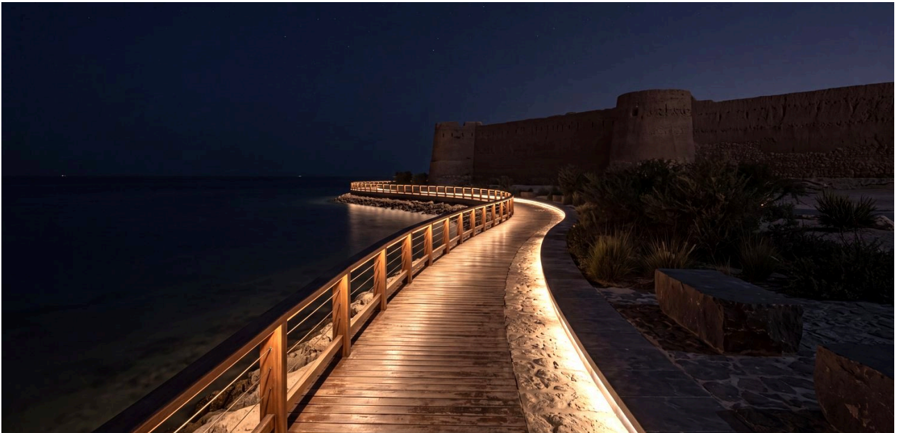
HANDRAIL-INTEGRATED LINEAR LIGHT ON A COASTAL BOARDWALK. THE WALKING SURFACE IS LIT, THE WATER AND THE SKY ARE NOT.
